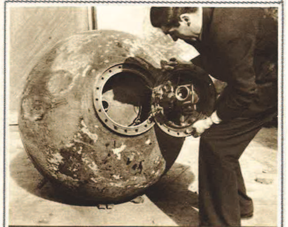
HOW THE BASQUES DEAL WITH INSURGENT MINES LAID OFF THEIR PORTS, SO MENACING BRITISH "BLOCKADE-RUNNERS": TAKING A MINE TO PIECES.
